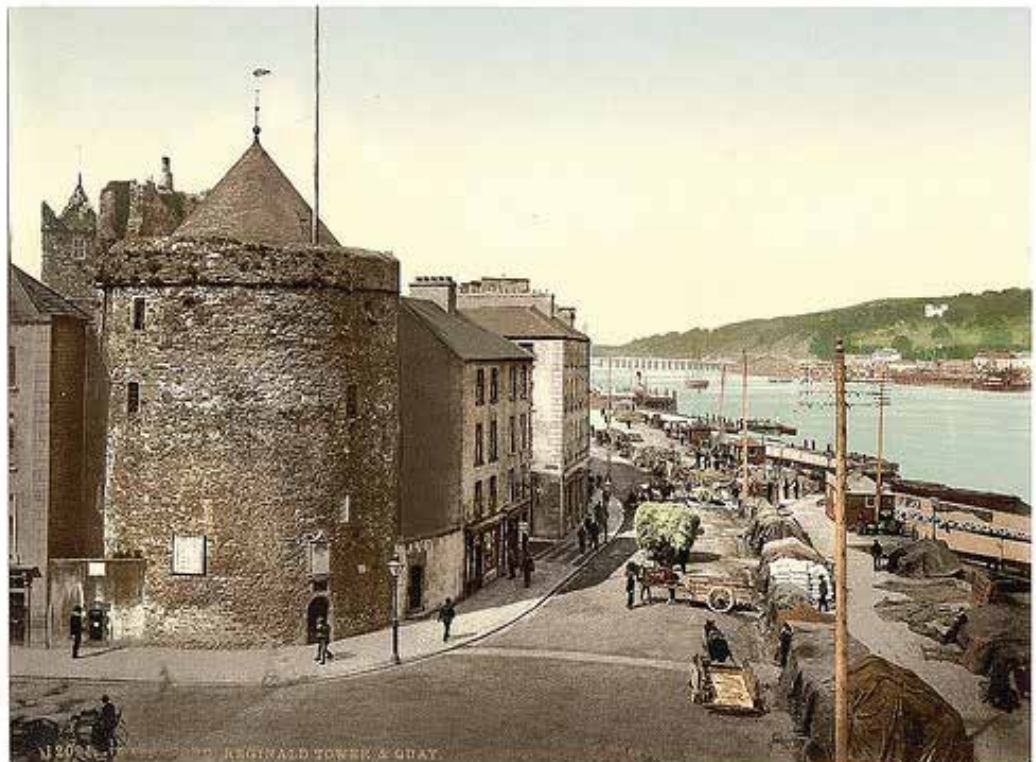
Reginald's Tower, Waterford, early twentieth century
